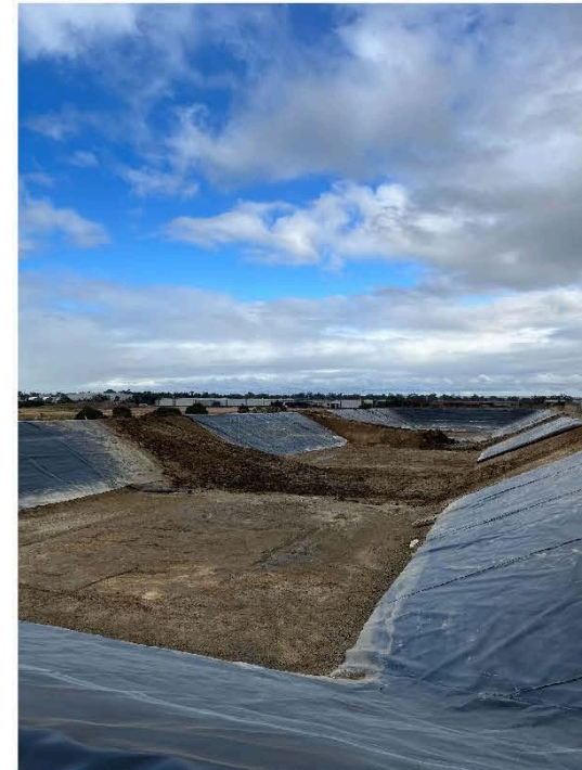
Early stages of the upkeep works includes stripping back the lining and removing the two soil bunds.
