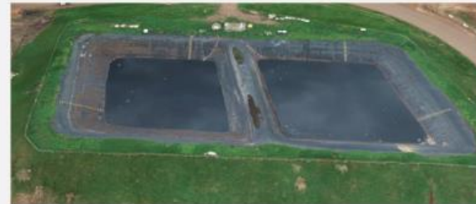
Ponds to be decommissioned before cell construction
