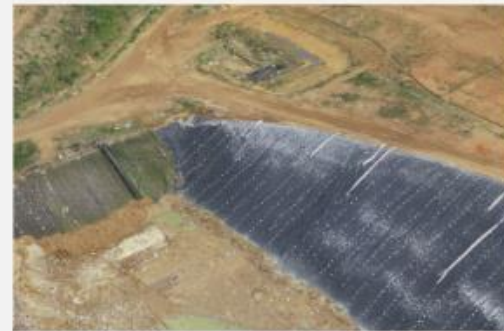
Sacrificial liner on wall of Cell 13
