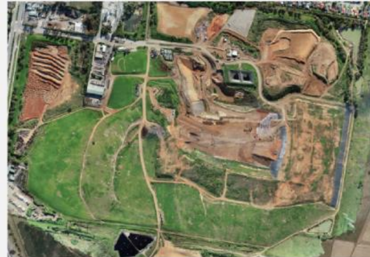
Overview of site - June
