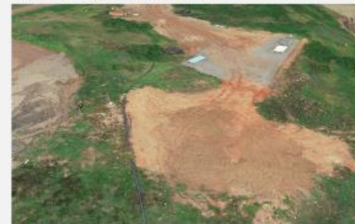
Material applied to Cell 3
