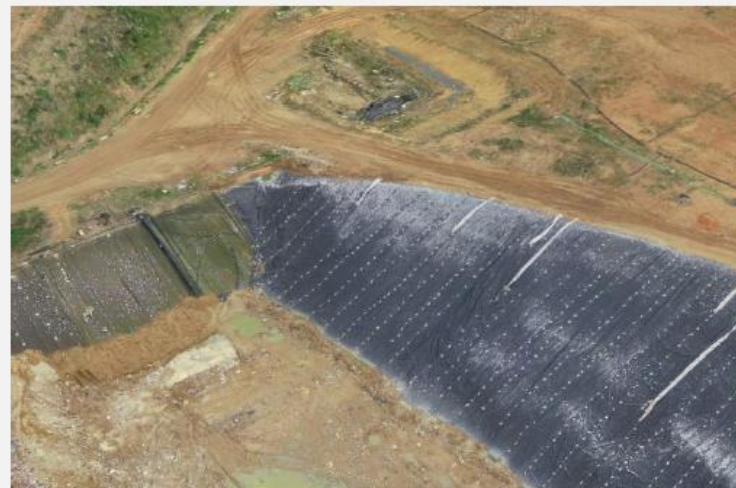
Sacrificial liner on wall of Cell 13
