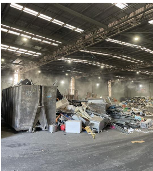
Photograph 3.1: Indicating the misting system used on site.
