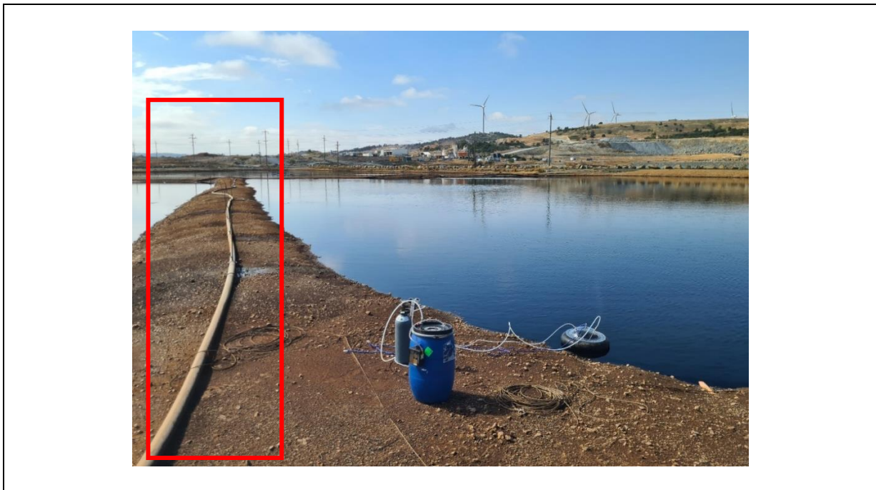
Photo 2.1 - A view of the ED3N middle bank spray evaporation system (outlined in red): 21 February 2023
