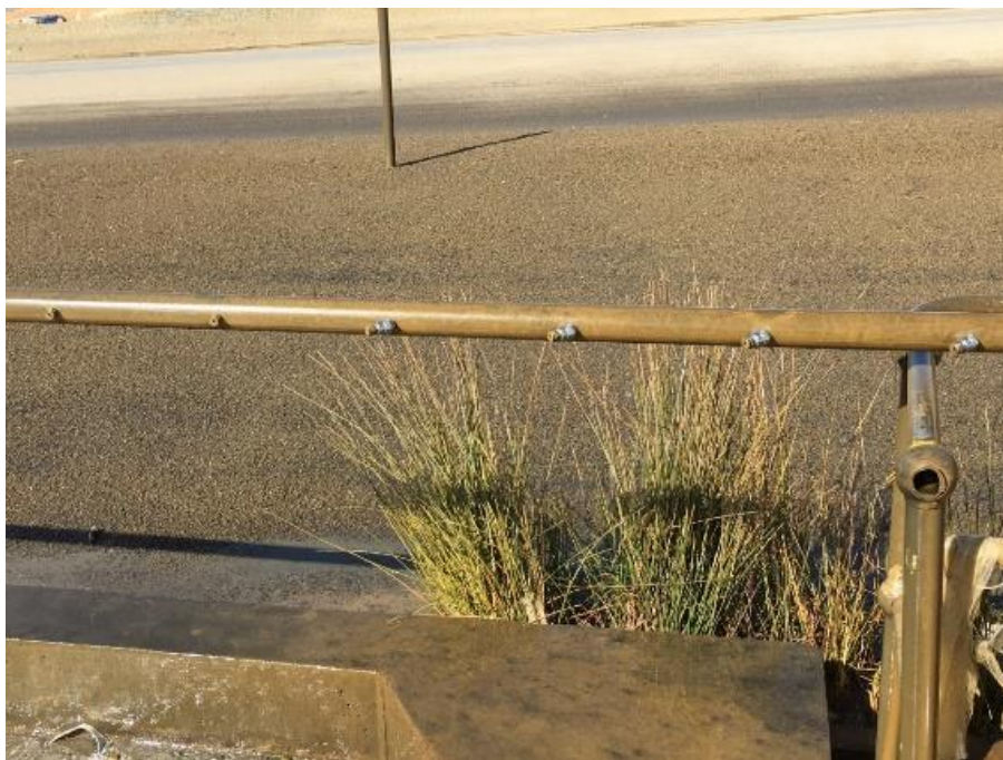
Photo 9.4 – Truck wash bay nozzle optimisation ( Source: 8 th IOA)
