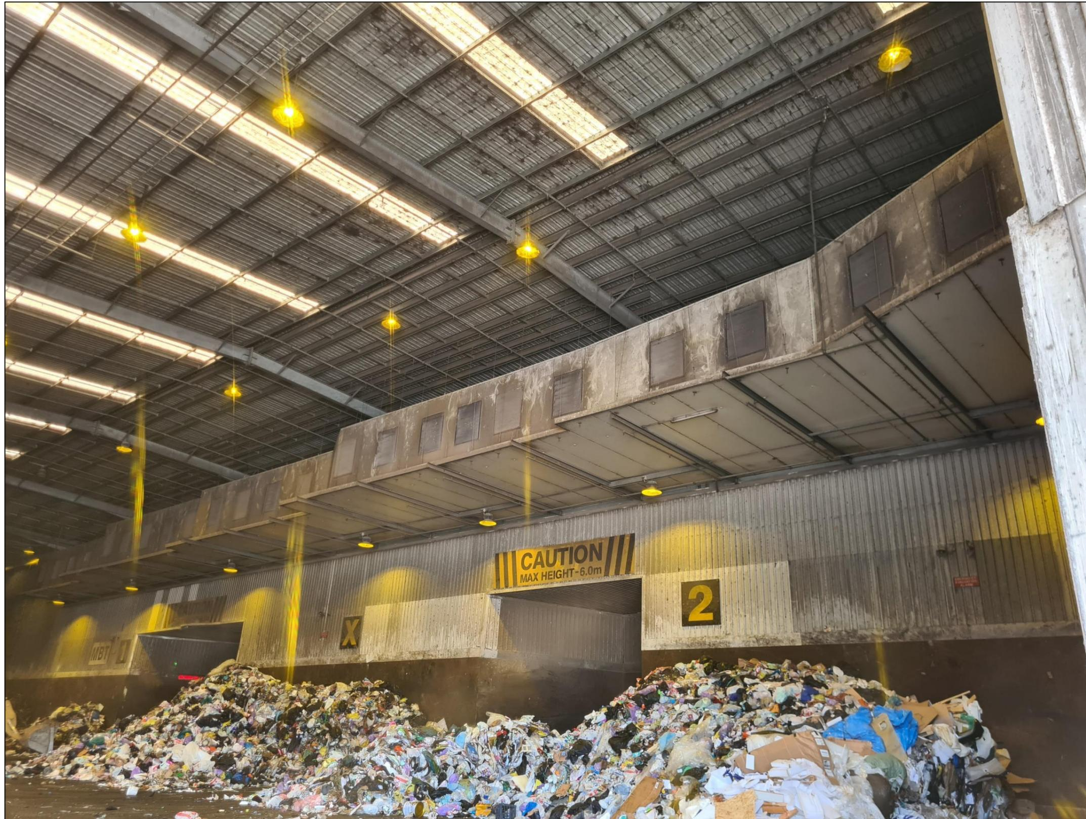
**Photo 4** – A view of the ventilation collection points: 21 December 2022 (Note: The collection grilles have an excess build-up of particulate matter)
