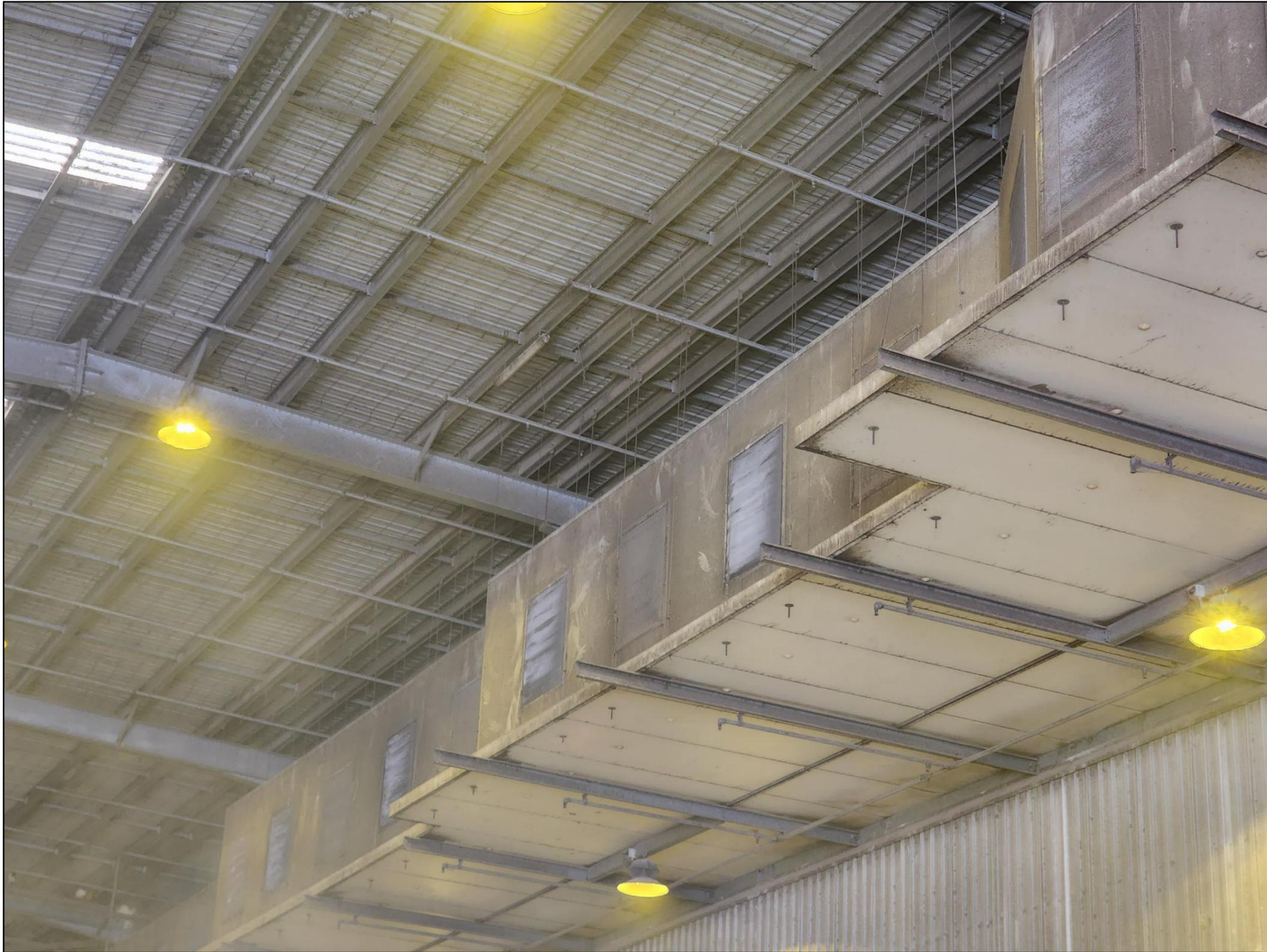
**Photo 4** – A view of the ventilation collection points: 1 June 2022 (Note: The collection grilles have an excessive build-up of particulate matter)
