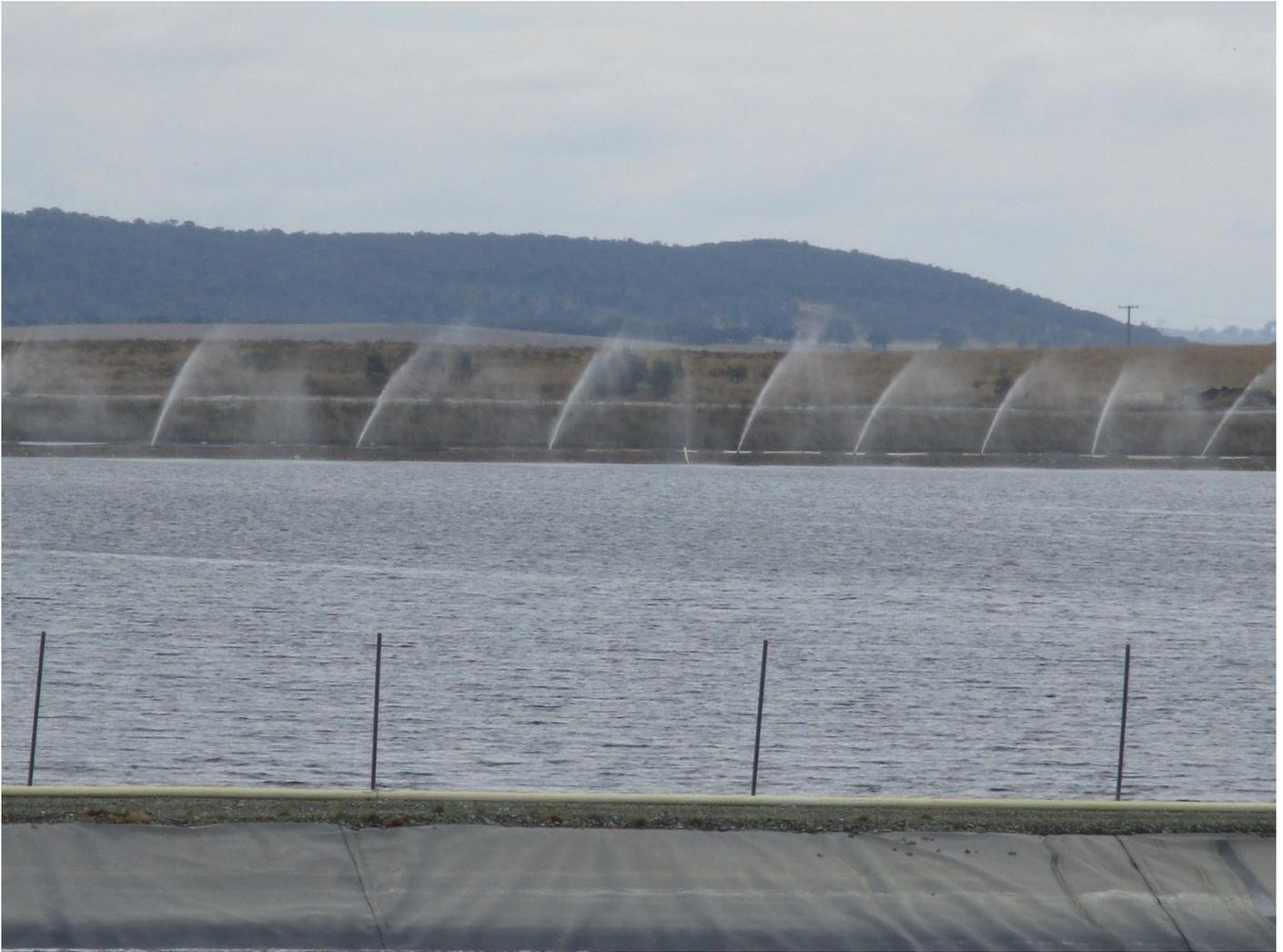
Figure B5. Photograph of treated leachate storage dam ED3N3 (foreground) and misting cannons in operation in ED3N4 (background).
