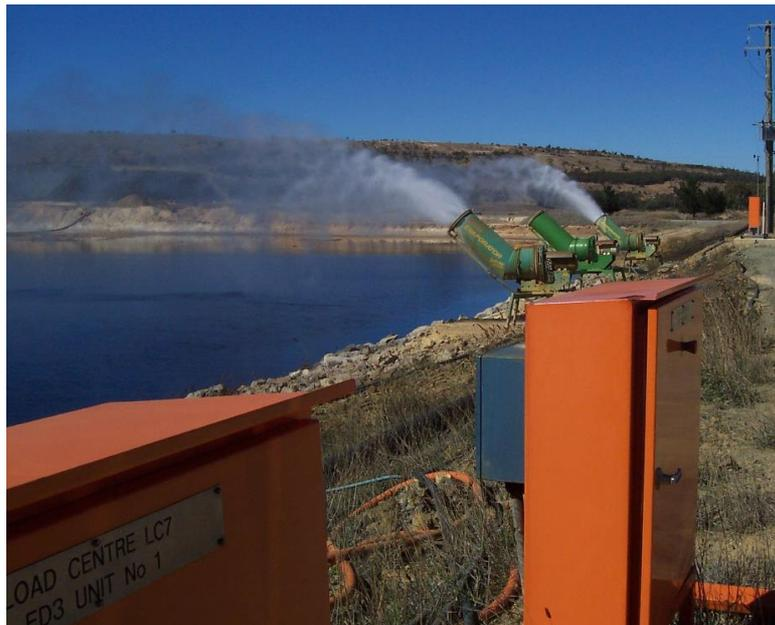
Figure 1: Evaporator units in action
