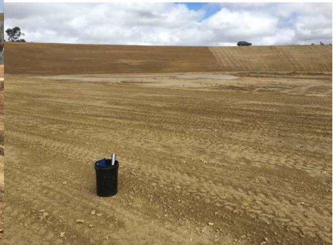
**Plates 3 & 4** (10 March 2016 & 5 February 2016). View over the northern end of ED3SS showing the access ramp used to transport clay materials (& remove waste rock) for the liner construction (completed with 0.3m capping of MBT). The completion of the insitu floor liner (i.e. 1.2 m) using reworked insitu clay-silt is shown (5 Feb 2016) before capping by MBT clay (0.3m thick).
