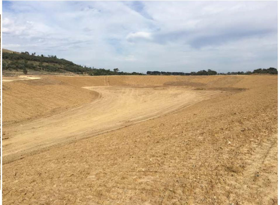
**Plates 1 & 2** (10 March 2016) Viewing south over the construction of ED3SS, showing completed batter slopes and floor levels (capped by 0.3m of MBT clay). Further compaction (smooth drum) and installation of the gravel layer (0.1m) is still in progress. The left plate shows the completed floor and walls and sampling location of ED3ss (F1= floor, blue bucket) and ED3SS (W1=wall).
