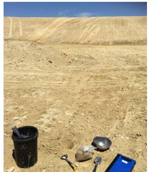
**Plates 1 to 5** (12 January 2016) Viewing north over liner construction works at ED3SS (use of D8, roller, excavator, water cart). An area of approximately 2500m<sup>2</sup> completed on SW corner to 0.9m thickness using re-worked and compacted weathered bedrock (siltstone) and clayey silt. Batter slopes completed using reworked insitu material (few meters thick). Two areas on the floor comprise hard rock which is removed and reused in the VOID.
