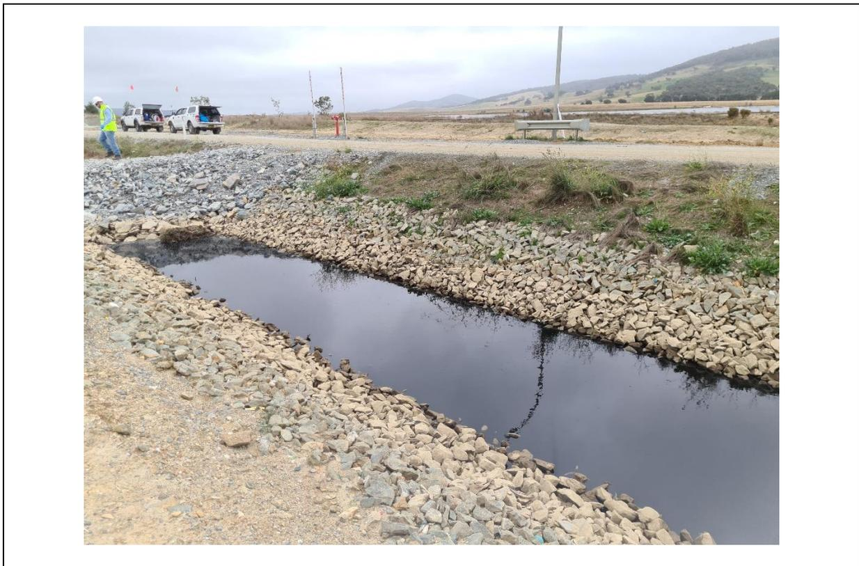
**Photo 2.6** – A view of the V-drain servicing the Maturation Pad at the MBT Facility: 24 March 2022
