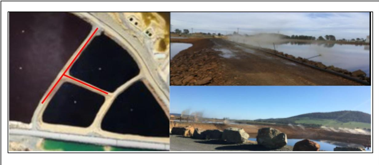
Figure 2.5 – The ED3N middle bank spray evaporation system (Source: WIP 2020)
