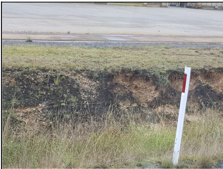
Photo 6: Eroded swale drain at the Crisps Creek IMF.
