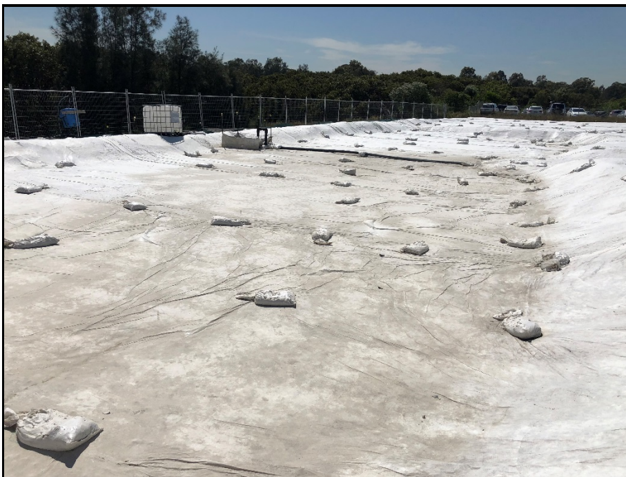
Photo 4: Temporary retention basin at northern end of the site.
