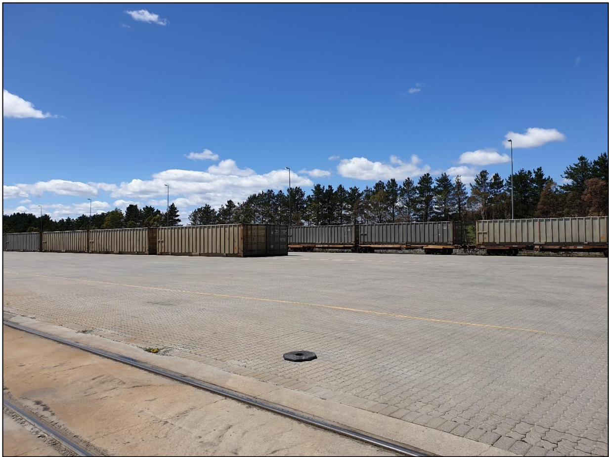
Photo 8.4 - The IMF facing south-east as observed during the Audit inspection visit on 20 February 2020
