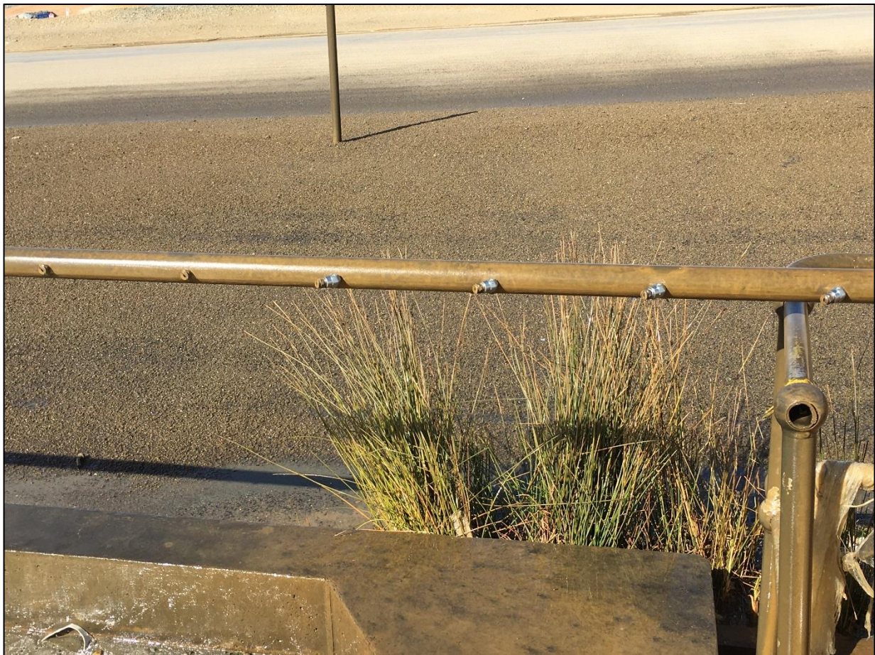
Photo 8.2 – Truck wash bay nozzle optimisation ( Source: Veolia)
