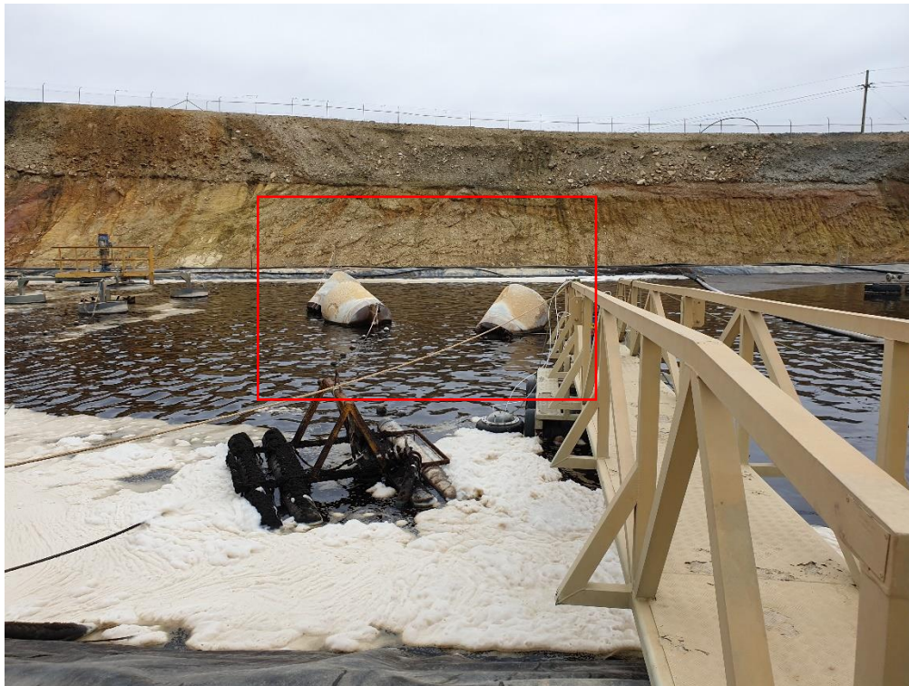
Photo 6.2 – The LTD on 18 February 2020 (highlighted area indicates location of aerator malfunction)
