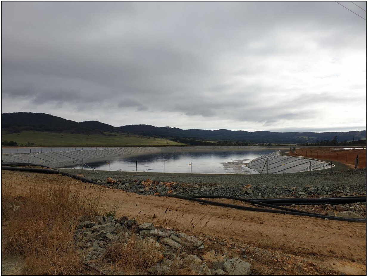
Photo 2.4 – ED1 Cofferdam: 18 February 2020
