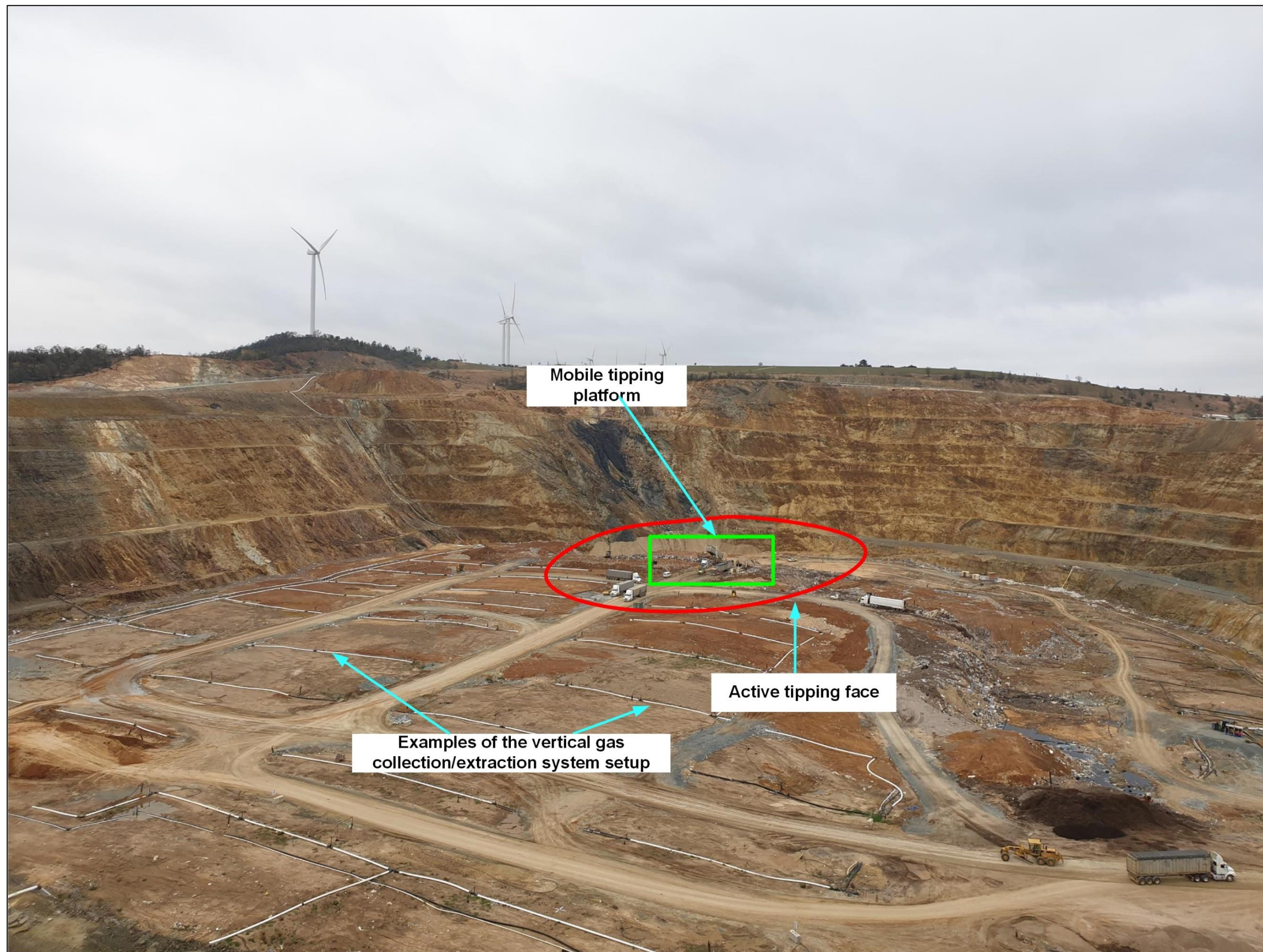
Figure 2.2 – Void layout and operations: 18 February 2020
