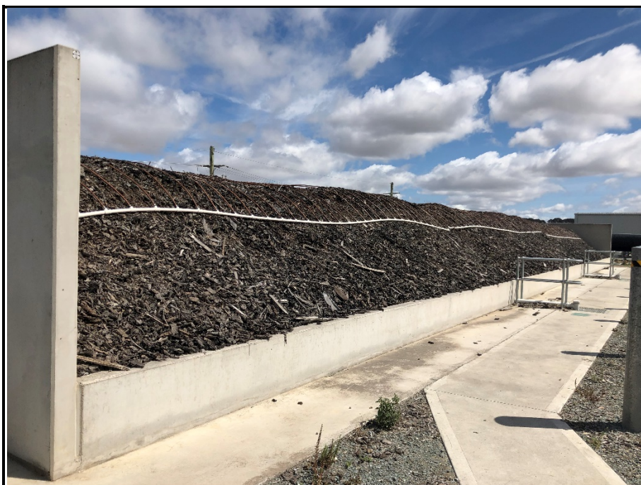
Photo 4: Biofilter located along the southern boundary adjacent to the administration building. Looking towards the west.
