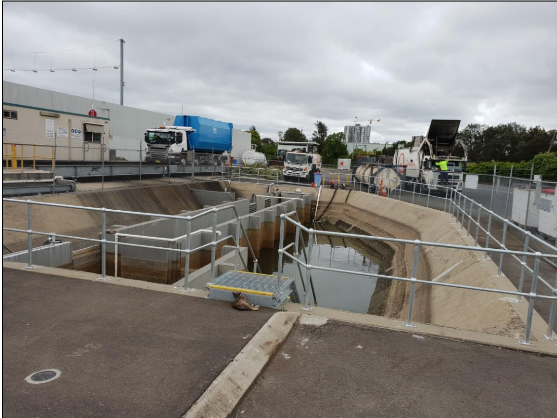
Photo 2.6 – Stormwater retention pond as found on 15 November 2018
