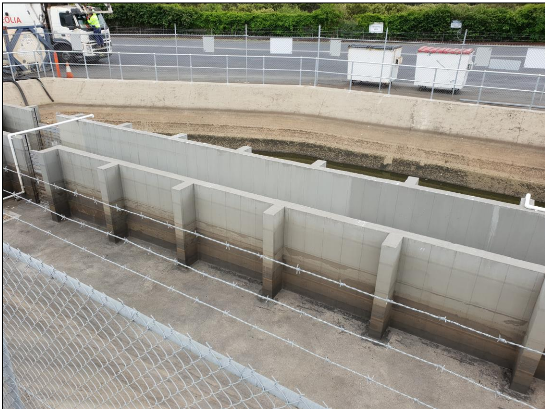
Photo 2.7 – Stormwater retention pond as found on 15 November 2018
