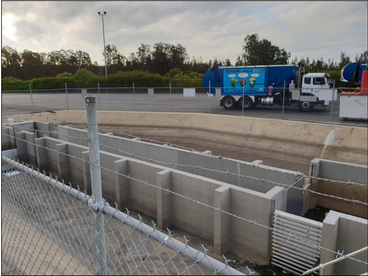
Photo 2.7 – Stormwater retention pond as found on 24 May 2018
