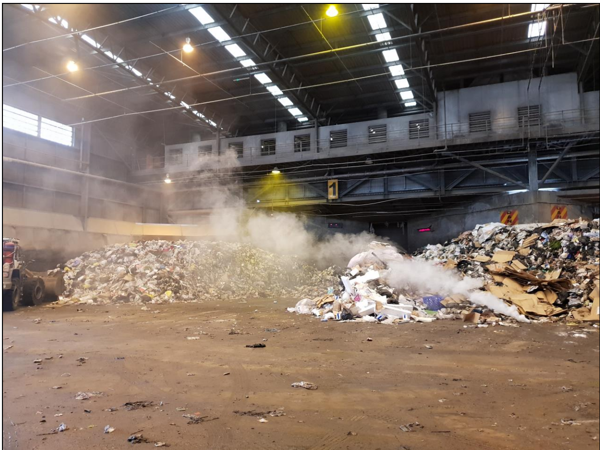
Photo 2.5 – Smoke testing within the TTB on 15 November 2018
