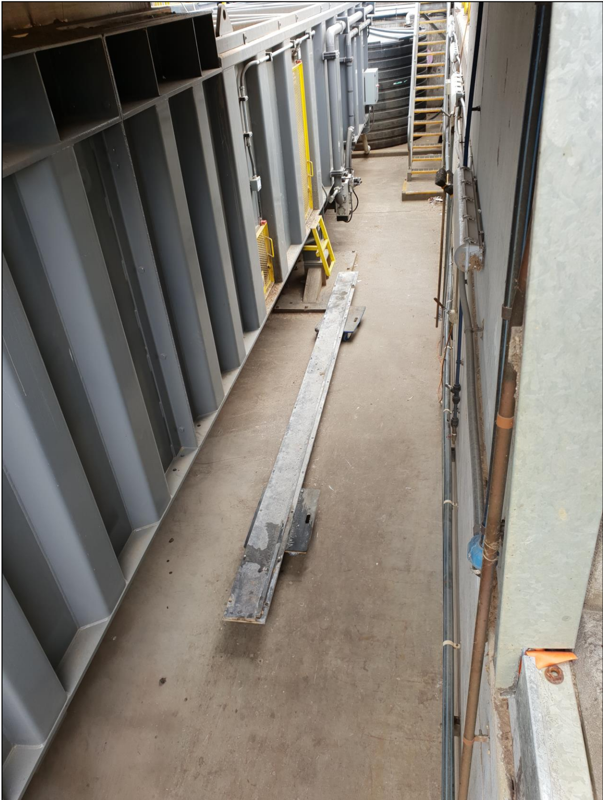
Photo 2.3 – Compactor area as found on 15 November 2018 (2 of 2)
