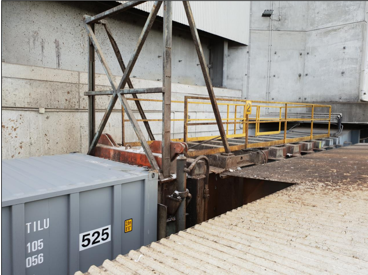
Photo 2.3 – Compactor area as found on 24 May 2018 (2 of 2)
