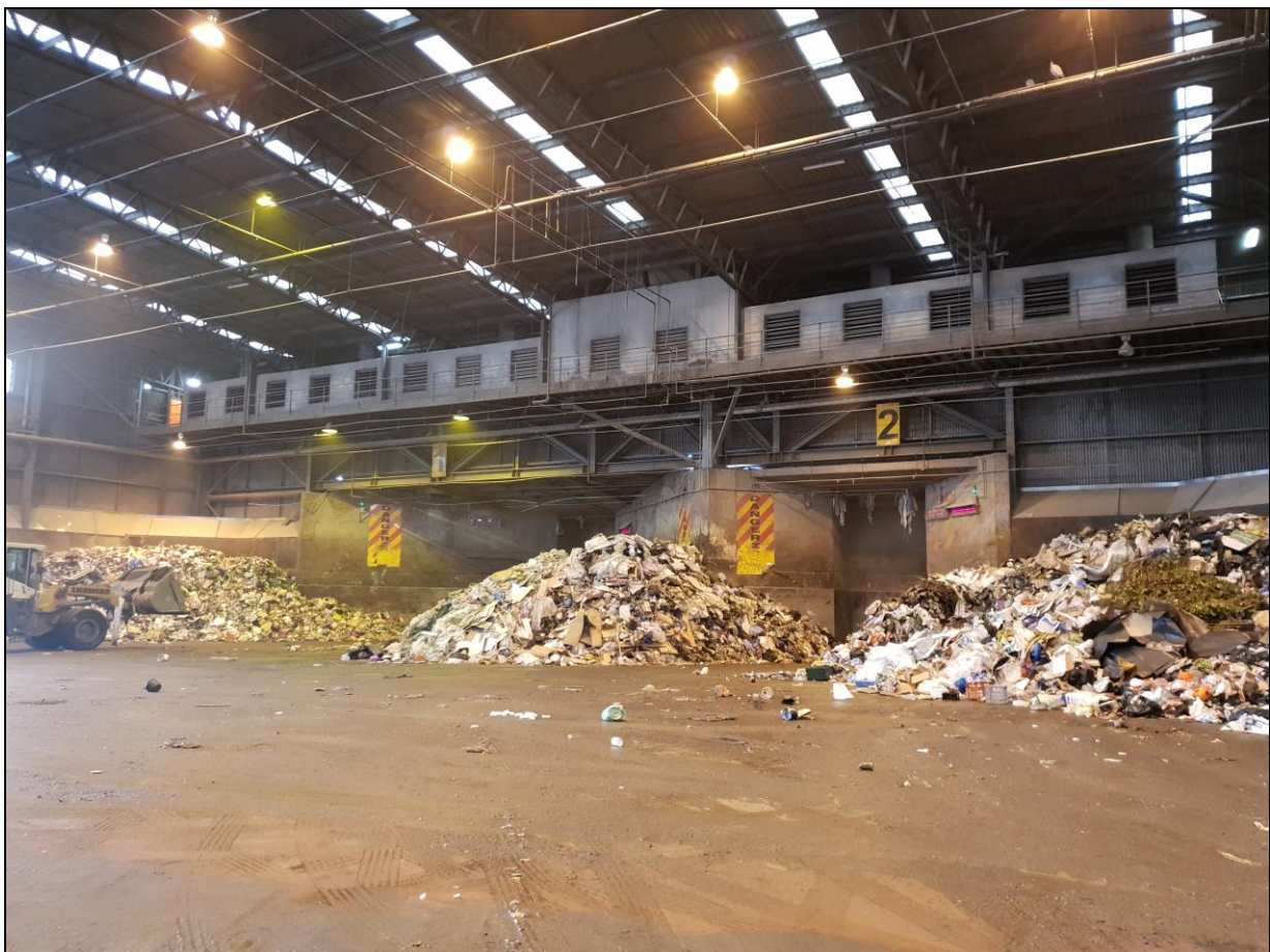
Photo 2.1 – Waste on-floor as found on 24 May 2018
