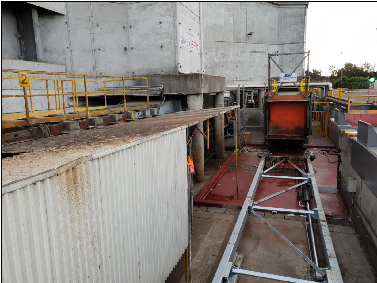
Photo 2.2 – Compactor area as found on 24 May 2018 (1 of 2)
