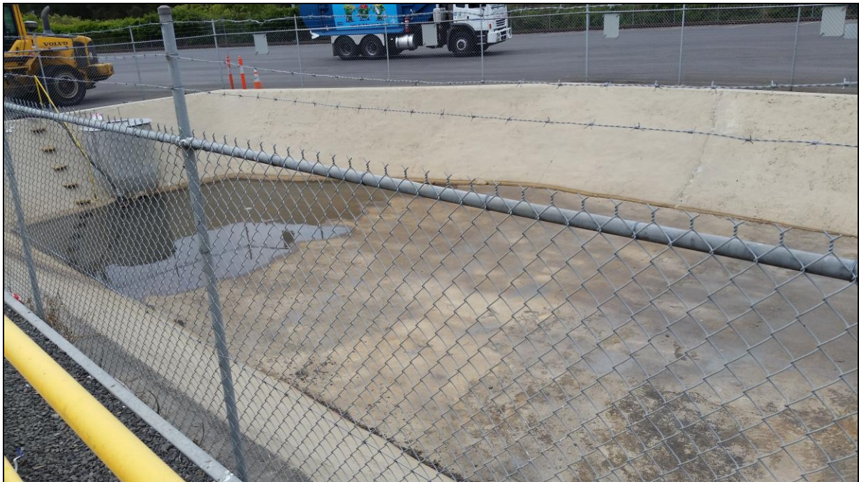
Photo 2.5 – Stormwater retention pond as found on 9 November 2016
