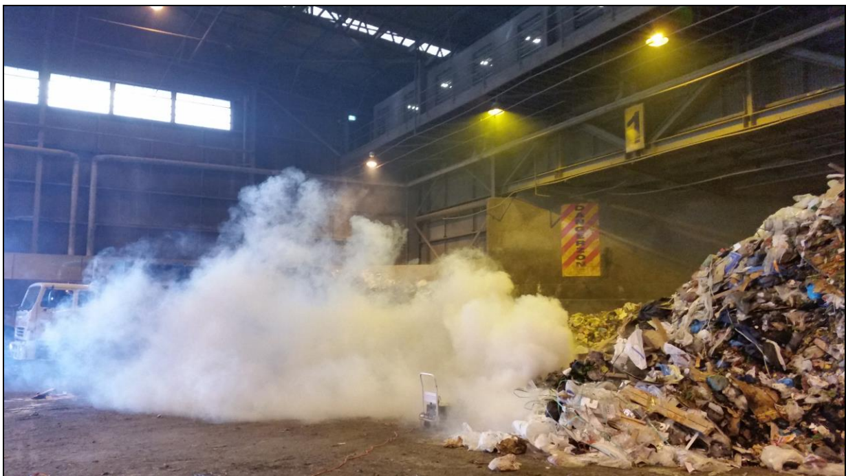
Photo 2.3 – Smoke testing within the TTB on 18 May 2016
