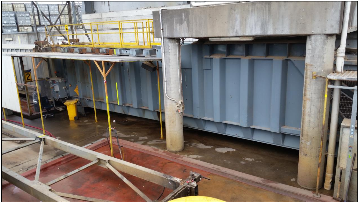
Photo 2.2 – Compactor area as found on 9 November 2016
