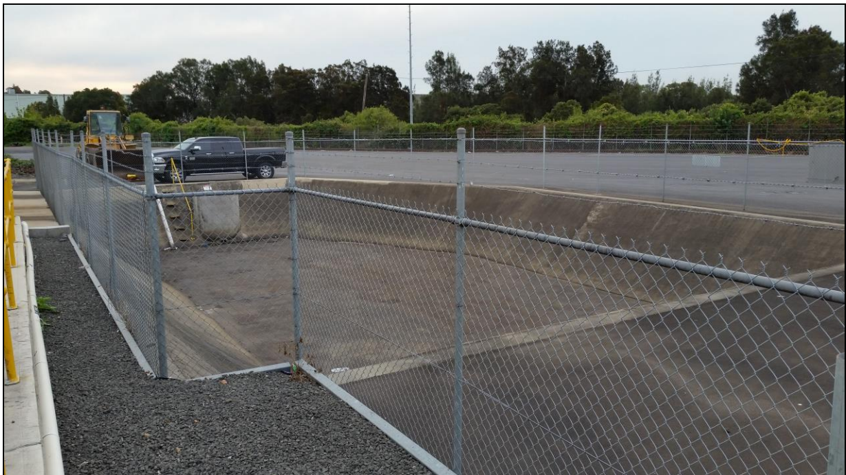
Photo 2.4 – Stormwater retention pond as found on 18 May 2016
